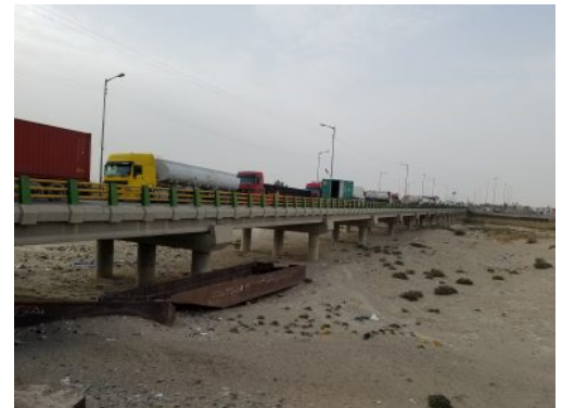
The bridge that links Afghanistan and Iran at Zaranj is too narrow, traffic builds up and inches across.
